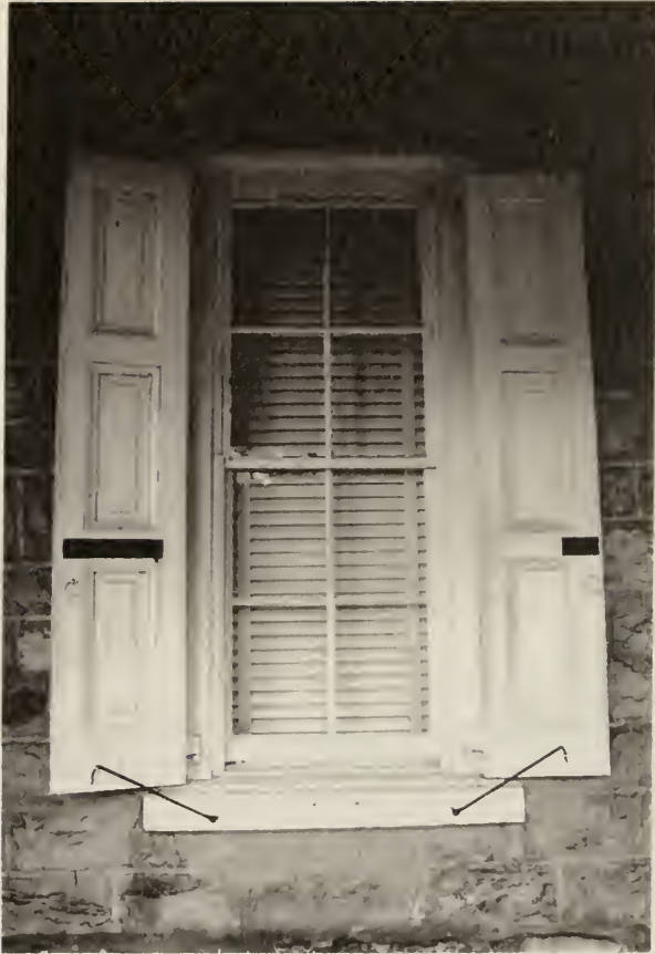
Figure 39. First floor window on south elevation of main section, illustrating an example of the type of window and shutters that were installed in the 1820s. (1994)
